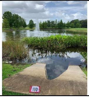
Recommendations & Notes: Minor erosion around mitered end pipes
