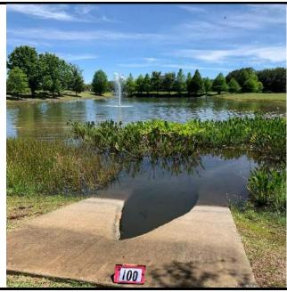
Recommendations & Notes: Minor erosion around mitered end pipes
