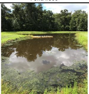
**Recommendations & Notes:** Yellow Boom needs removed. This Turbidity Boom was put here for the initial stages of land clearing.
