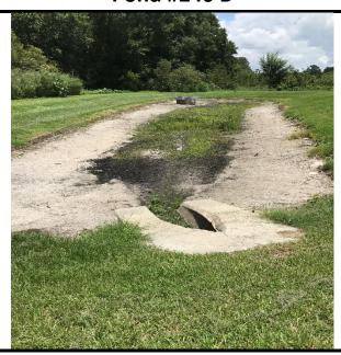
Recommendations & Notes: Will keep an eye on the concrete cap minimal undermining to insure it does not crack. We can provide a proposal for this (same).
