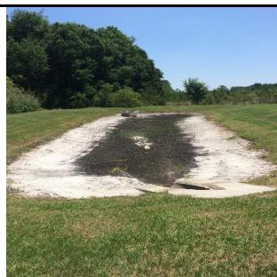
Recommendations & Notes: Will keep an eye on the concrete cap minimal undermining to insure it does not crack. We can provide a proposal for this (same).
