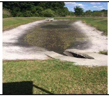
Recommendations & Notes: Will keep an eye on the concrete cap minimal undermining to insure it does not crack. We can provide a proposal for this (same).
