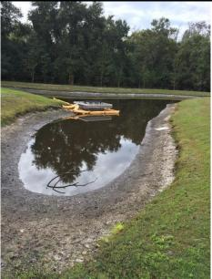
**Recommendations & Notes:** The missing grate on the control structure has been replaced on this pond.
