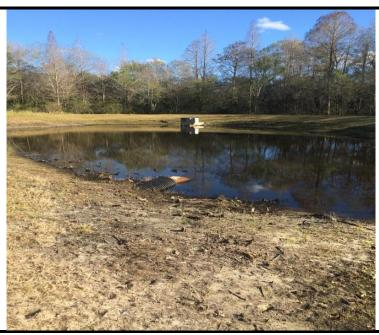
**Recommendations & Notes:** Also, the drain pipe inlet in this pond is more than 50% full of sediment & needs maintenance.
