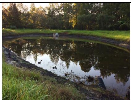
**Recommendations & Notes:** Also, the drain pipe inlet in this pond is more than 50% full of sediment & needs maintenance.
