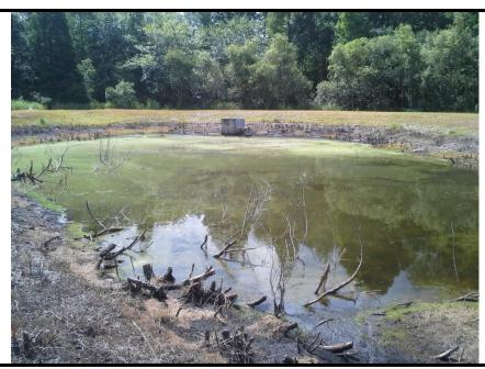
**Recommendations & Notes:** Now would be a good time to remove the sticks & stumps when water levels are low. Even though this pond is mostly out of site. Also, the drain inlet in this pond is more than 50% full of sediment & needs maintenance.
