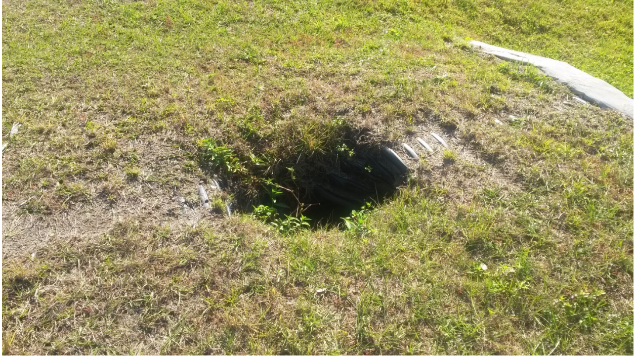
Failed storm pipe near pond 220
