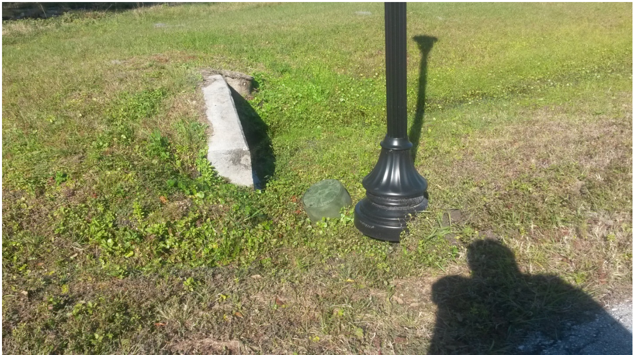
Erosion under the street light and valve box
